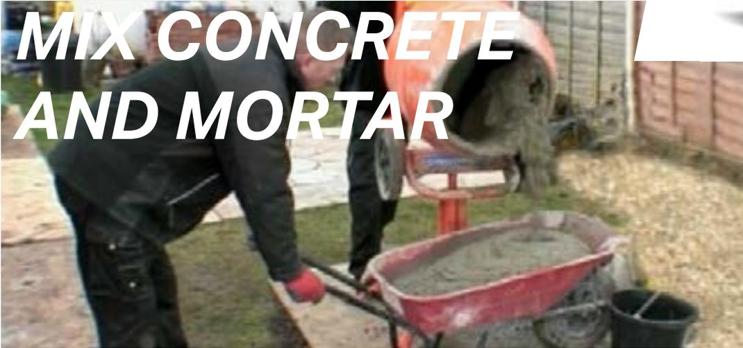
When mixing concrete or mortar, accurate proportioning or gauging of materials and thorough mixing are essential. Using a shovel to measure out the different constituents is not accurate enough and can lead to problems and variability in performance, the use of batch boxes or other containers is strongly recommended. Use the same size container for measuring all materials. A heavy duty 15 litre bucket is a convenient size, always use a separate bucket and shovel for cement.
